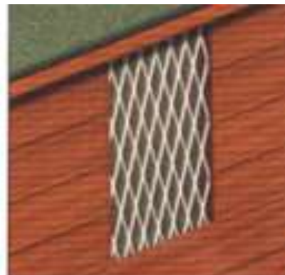
Internal diamond mesh grille over shed window
